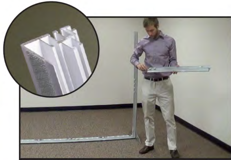
Insert CSS halfway into upper right extrusion and tighten 2 thumb screws. Mitre edge will be on top.
