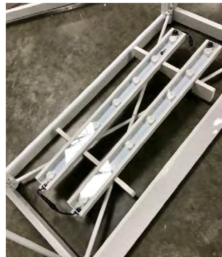
Completed rows of light bars
