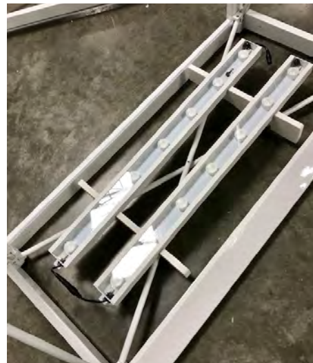
Completed rows of light bars
